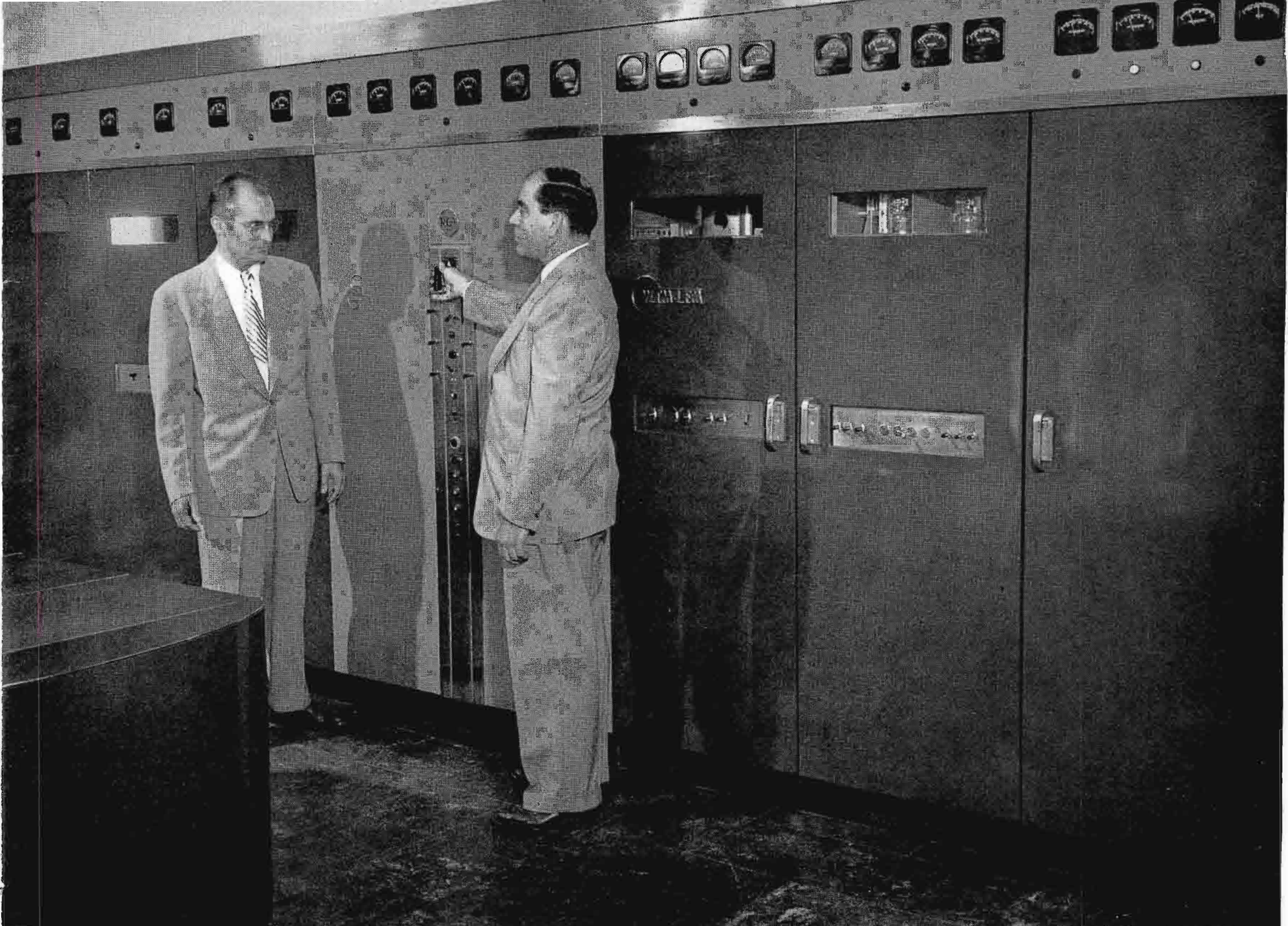
FIG. 2 (above). Phillip B. Laeser, WTMJ chief engineer, observes as W. B. Fletcher, RCA engineer, demonstrates ease of power cut-back to 10 KW from 50 KW operation. All units of the RCA 50 KW FM transmitter are mounted behind a unified front panel providing a neat business-like arrangement with complete accessibility.
