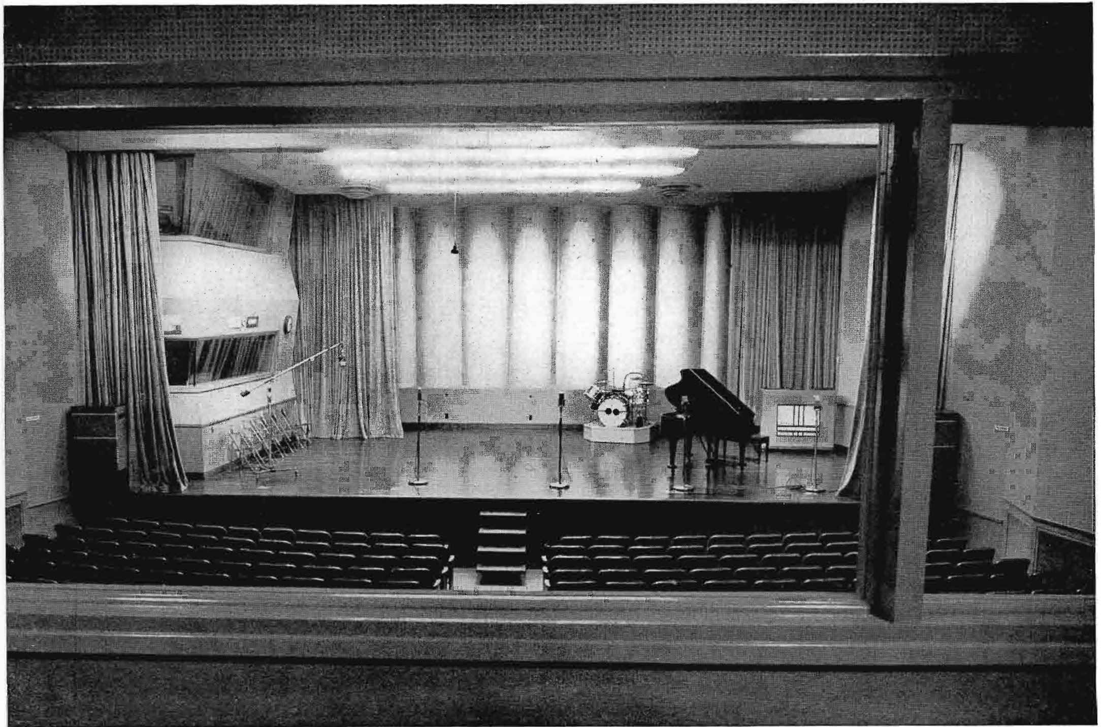
▲ FIG. 5. This is one of CMQ's huge theatre-type studios which seats 350 people. Its large stage can accommodate a full 150-piece symphony orchestra. On either end of the stage can be seen an RCA LC-1A Loudspeaker which is part of the sound reinforcement system for the studio. On the left side of the stage is the engineer's control booth and immediately above it is the sponsor's booth.
