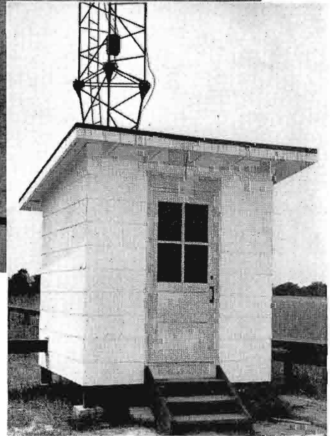
FIG. 6. Four guyed 400-foot towers arranged in a square make up the station's directive antenna array. Phasing equipment for the towers is housed alongside the 10 KW transmitter in a matched panel. The enclosure is standard RCA equipment which is added to transmitters when phasing equipment is employed. Inset shows one of the tower houses located at base of each antenna tower.
